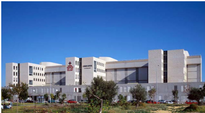
Hospital San Juan Alicante Laboratorios CORE
